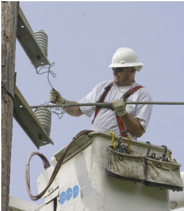
Figure 8.7 Line workers are required to adhere to approach minimums and inadvertent movement allowances.
